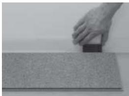
**2. Fix the first floor board in place with distance spacers (keep expansion gap of 10-15 mm around perimeter). Always align the boards with the tongue side parallel to the wall.**
