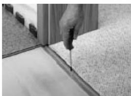
**7. In doorways, mount a suitable transition moulding system to ensure the necessary expansion space. Leave an expansion space of approx. 5 mm between the board and the base section of the moulding.**
