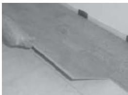
**5. The remaining rows should be installed board by board. First, the board is angled into the previous row along the long side by applying a small amount of force.**
