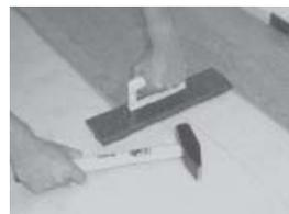
**6. Then you interlock the board with the board to its left at the short side, using hammer and tapping block or, in hard-to-reach areas, the pull tool. Ensure that the joints are staggered with at least 30 cm difference.**
