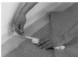
**8. Cut to size and fit in the boards of the last row. Leave a gap of 10 to 15 mm between the boards and wall.**
