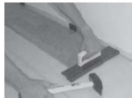
**3. Join the panels of the first row at the short sides rotating to fit into one another or using hammer and tapping block.**
