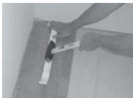
**4. Measure the last board of the first row and keep in mind to leave the expansion gap between the board and the wall. Cut the board to size and fit it in with the pull tool. Start the second row with the leftover piece of the first row.**
