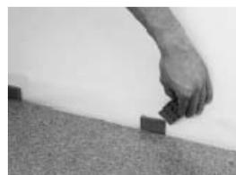
**9. Remove all distance spacers. Fasten skirtings (with or without clip system) to the walls.**
